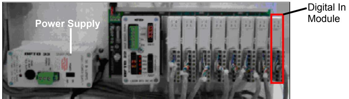
Figure 7-8: Element Monitor Controller
