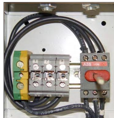
Figure 1-18 Disconnect Switch and Power Connection Terminal Blocks
