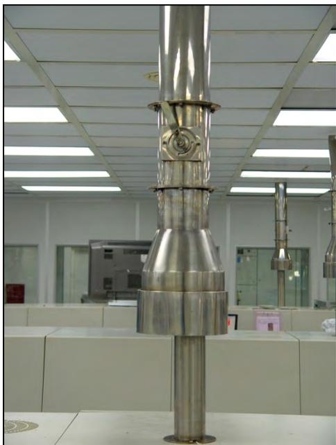
Figure 1-24 Exhaust Connection
