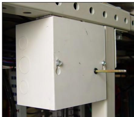
Figure 1-16 Interlock Disconnect Switch Enclosure
