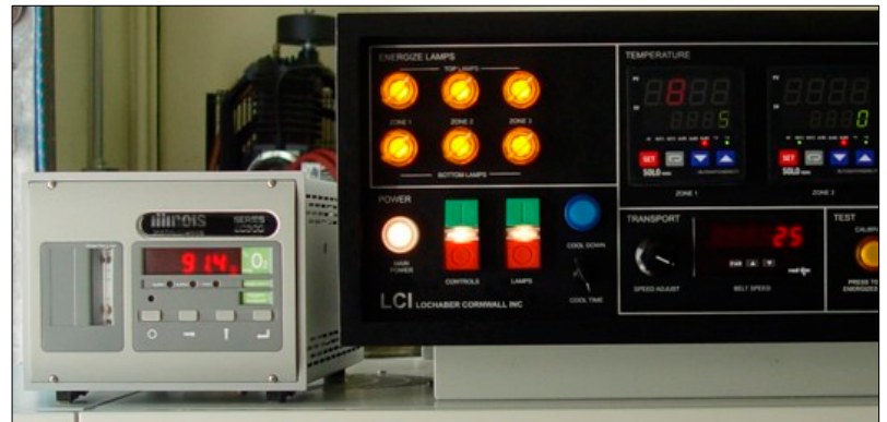
Figure 6-10 Oxygen Analyzer next to Control Console
