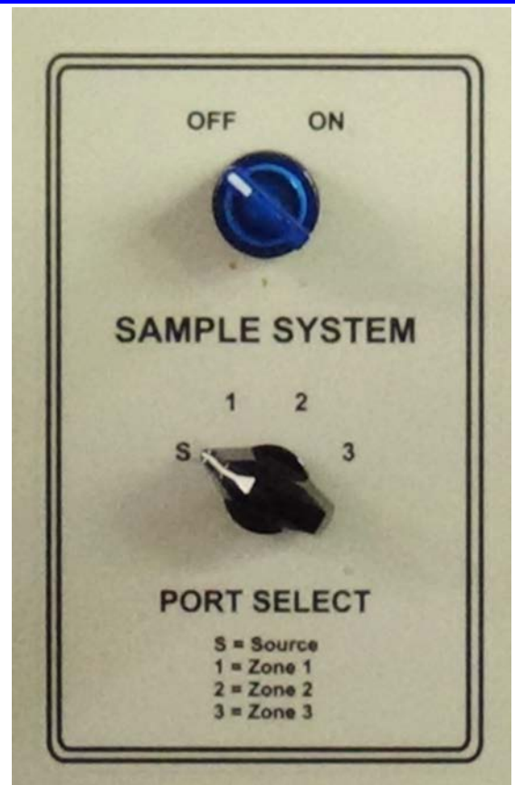
Figure 6-12 Sample System control panel (shown with Supply Gas Mixing System)
