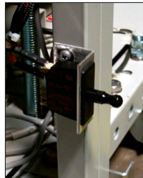
Panel Switch Installed - Bypass (out) Position
