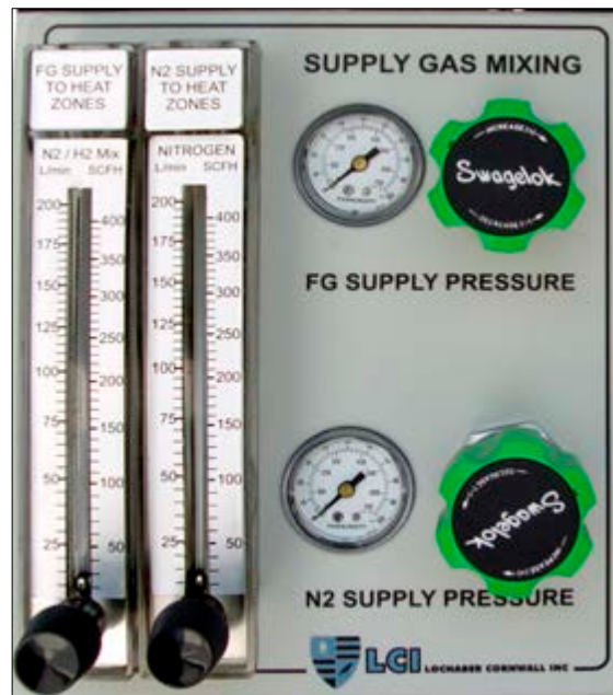
Figure 6-7 Supply Gas Mixing System Control Panel
