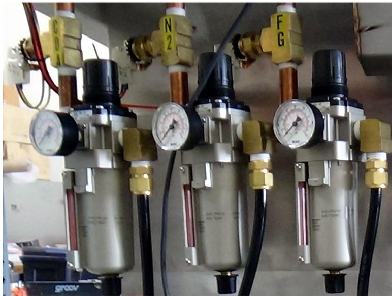
Figure 1-10 Filter regulators in furnace enclosure
