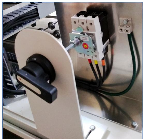
Figure1-25 3-Ph Circuit Breaker-Panel OFF
