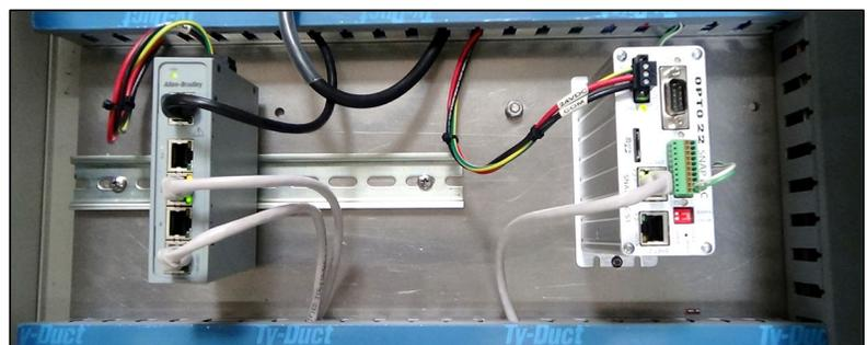
**Figure 1-17 Ethernet Switch (L) & Controller (R)**
