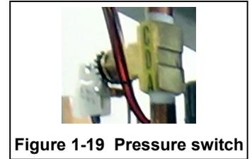
Figure 1-19 Pressure switch
