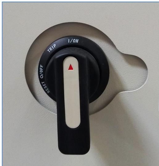
Figure 1-24 3-Phase Circuit Breaker
