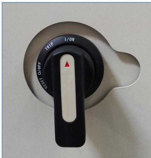
Figure 1-24 3-Phase Circuit Breaker
