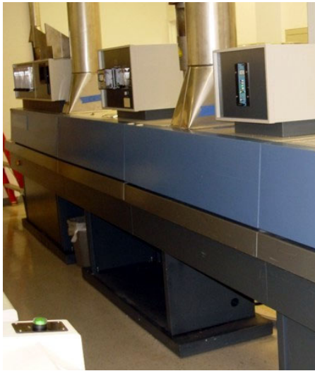
Figure 1-33 Cabinet Exhaust Example
