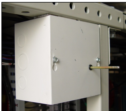
Figure 1-21 Interlock disconnect switch enclosure
