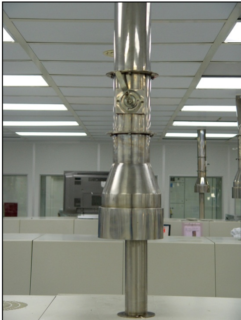
Figure 1-31 Exhaust Connection
