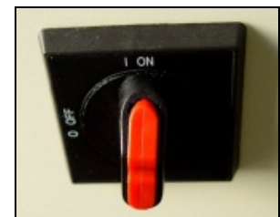
Figure 1-20 Interlock Disconnect switch
