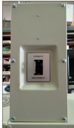
Figure 1-18 Circuit Breaker enclosure
