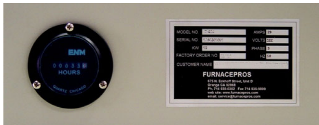
Figure 1-16 Elapsed Time Meter and Nameplate
