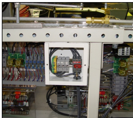
Figure 1-22 Enclosure, cover removed
