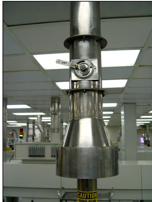
Figure 1-32 Exhaust Connection Detail
