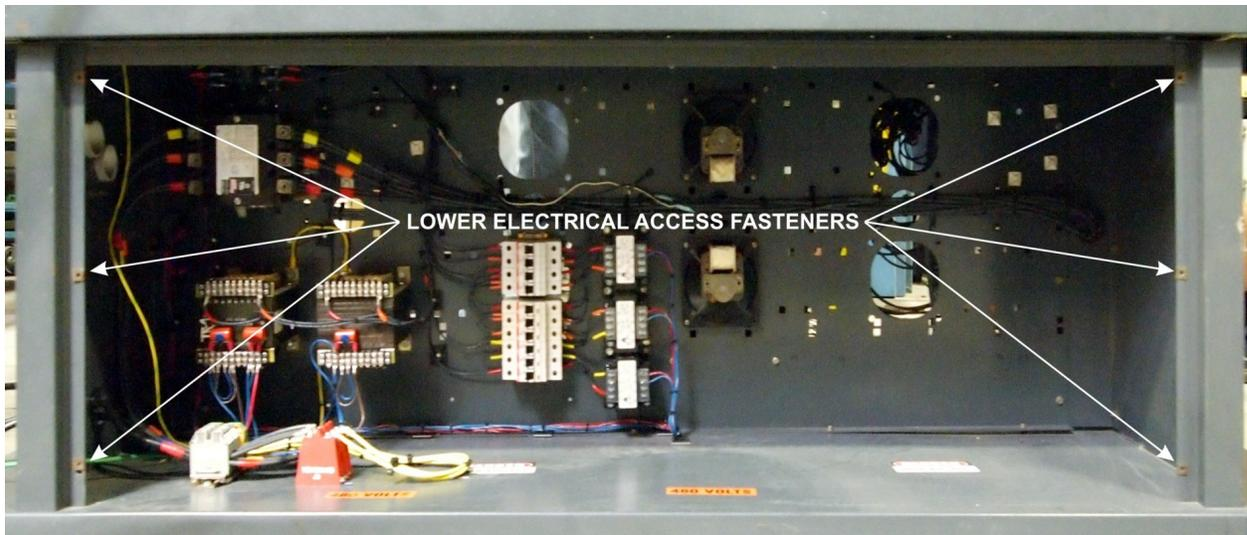
Figure 4-5 Lower Electrical Panel access
