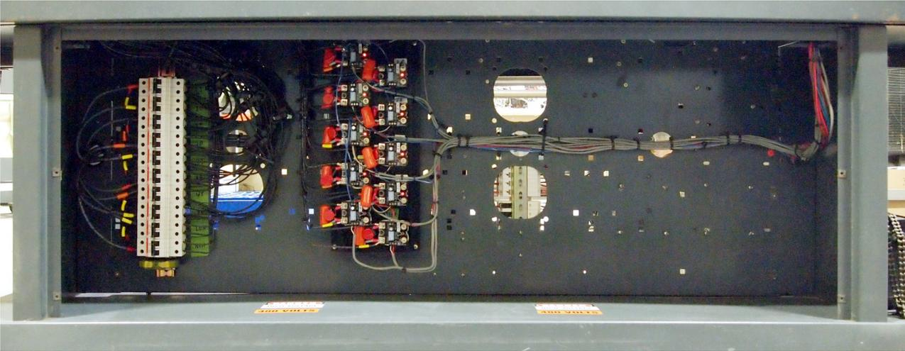
Figure 4-10 SCR Panel with EM sensors
