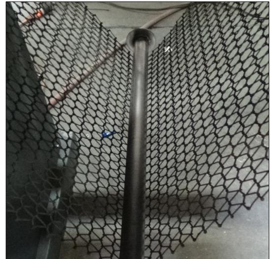
Figure 4-31 Proper Alignment of Belt Weight
