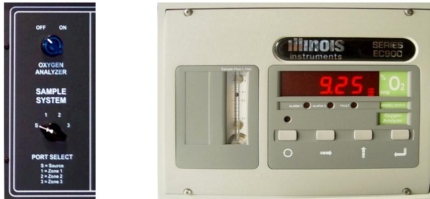
Figure 4-55 OSS Sample System Panel & Oxygen Analyzer
