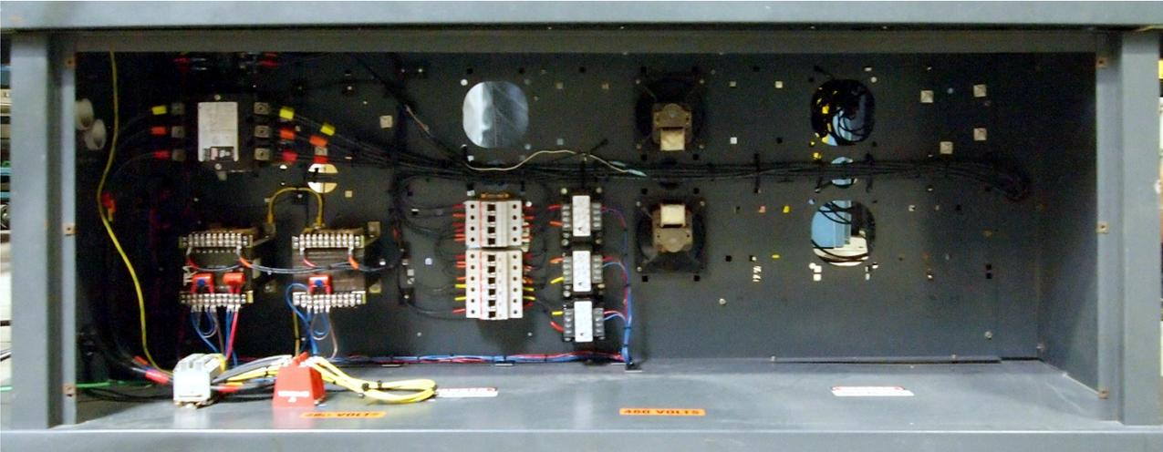
Figure 4-9 Power Distribution and Safety panels
