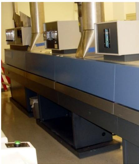
Figure 2-35 Cabinet Exhaust Example
