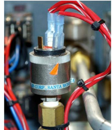
Figure 2-46 Pressure Switch
