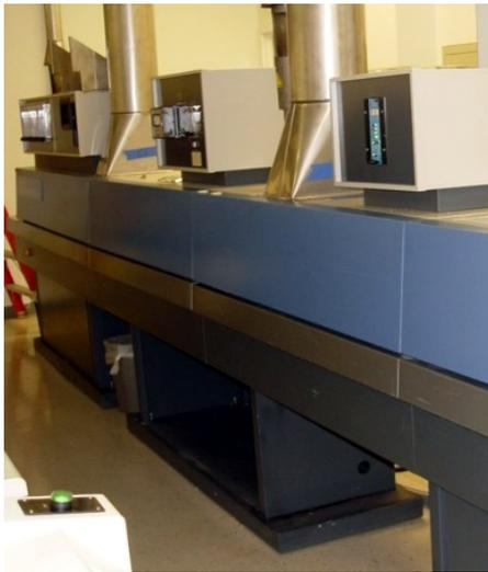
Figure 2-35 Cabinet Exhaust Example
