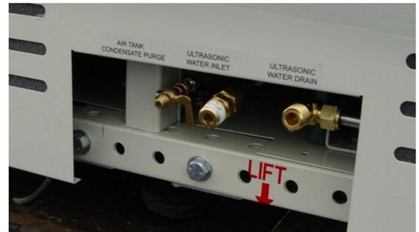
Figure 2-44 UCD Water Connections and Air Purge (Reservoir option only)
