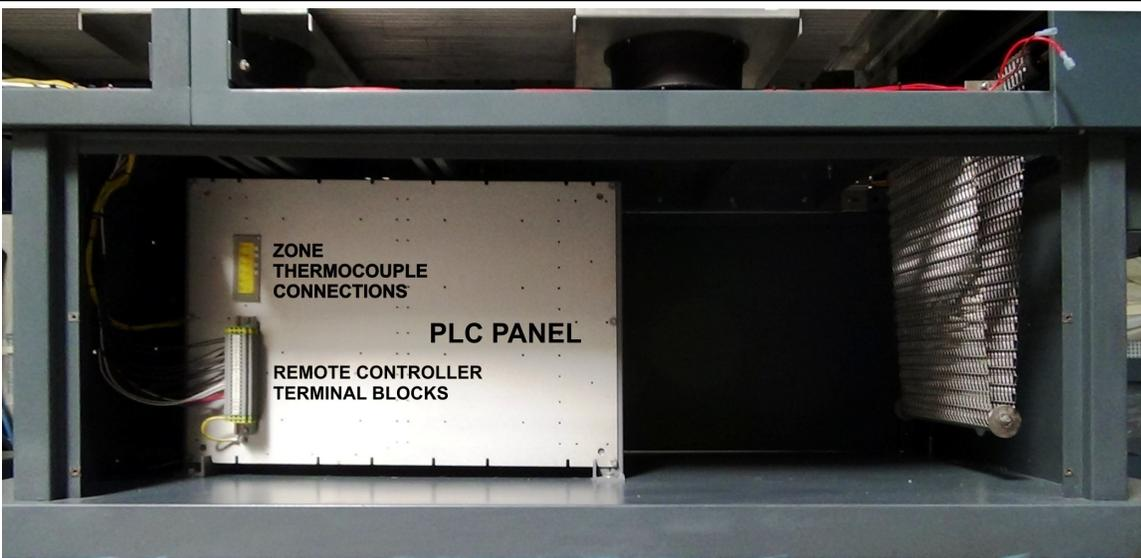
Figure 2-43 PLC Panel and Remote Connections
