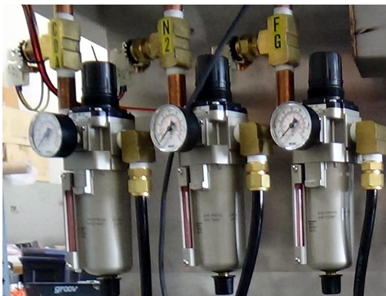
**WARNING: The flowmeters on these furnaces are rated at 70 psi (5 bar) maximum. Operating above 70 psi exposes the operator to possible injury, may cause damage to the furnace internals and insulation and voids the furnace warranty.**
