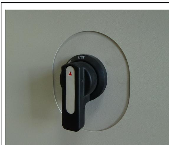
Figure 0-21 3-Phase Circuit Breaker
