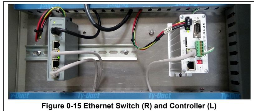
Figure 0-15 Ethernet Switch (R) and Controller (L)
