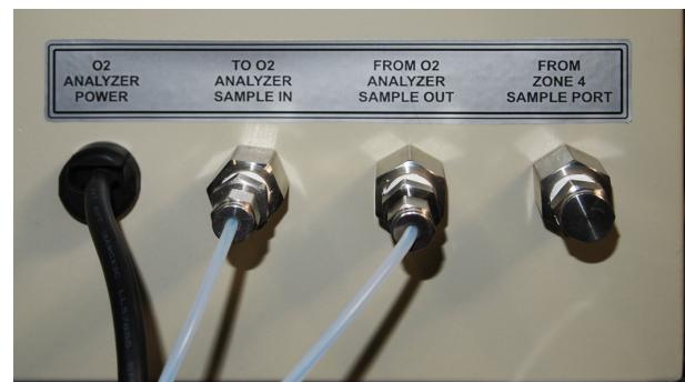
Figure 2-33 OA furnace control enclosure connections
