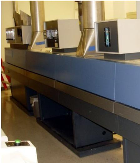
Figure 2-27 Cabinet Exhaust Example
