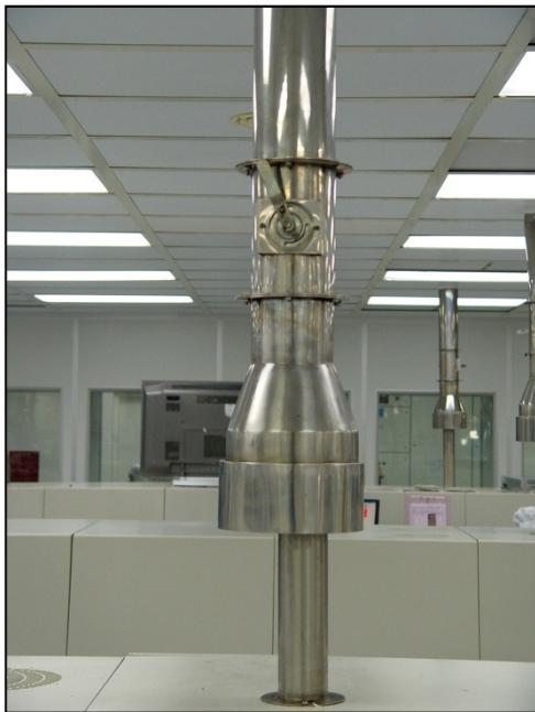
Figure 2-25 Exhaust Connection
