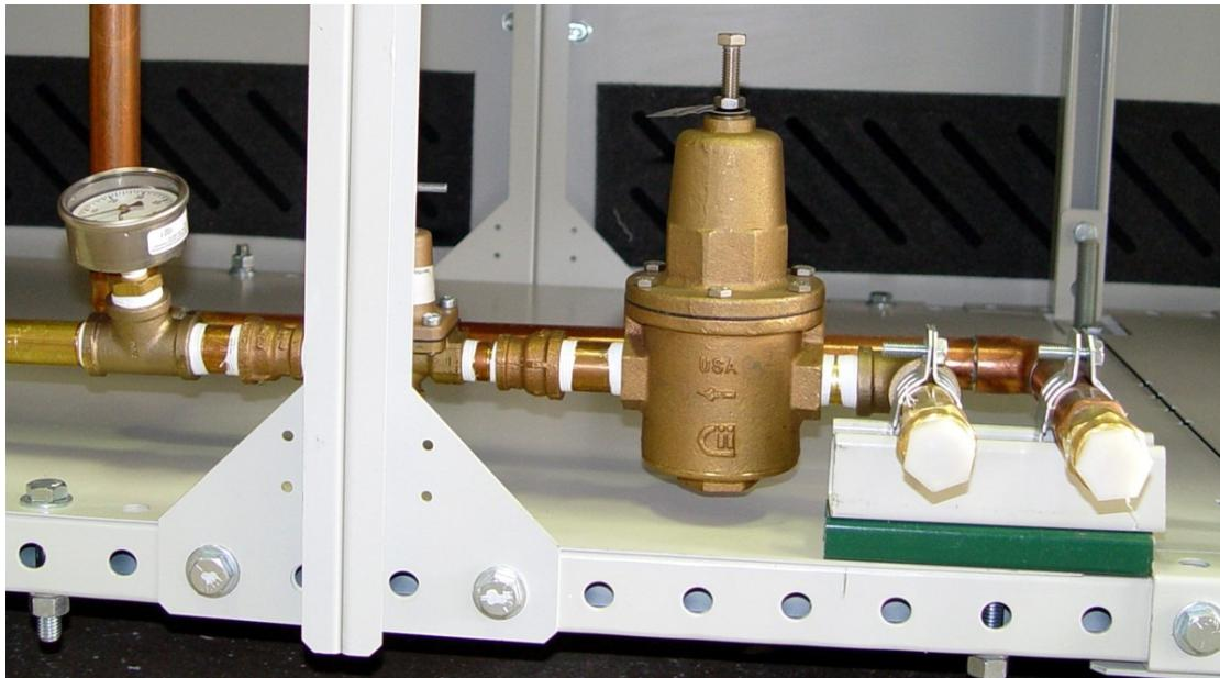
Figure 2-36 CAWC Water Supply & Drain Connections
