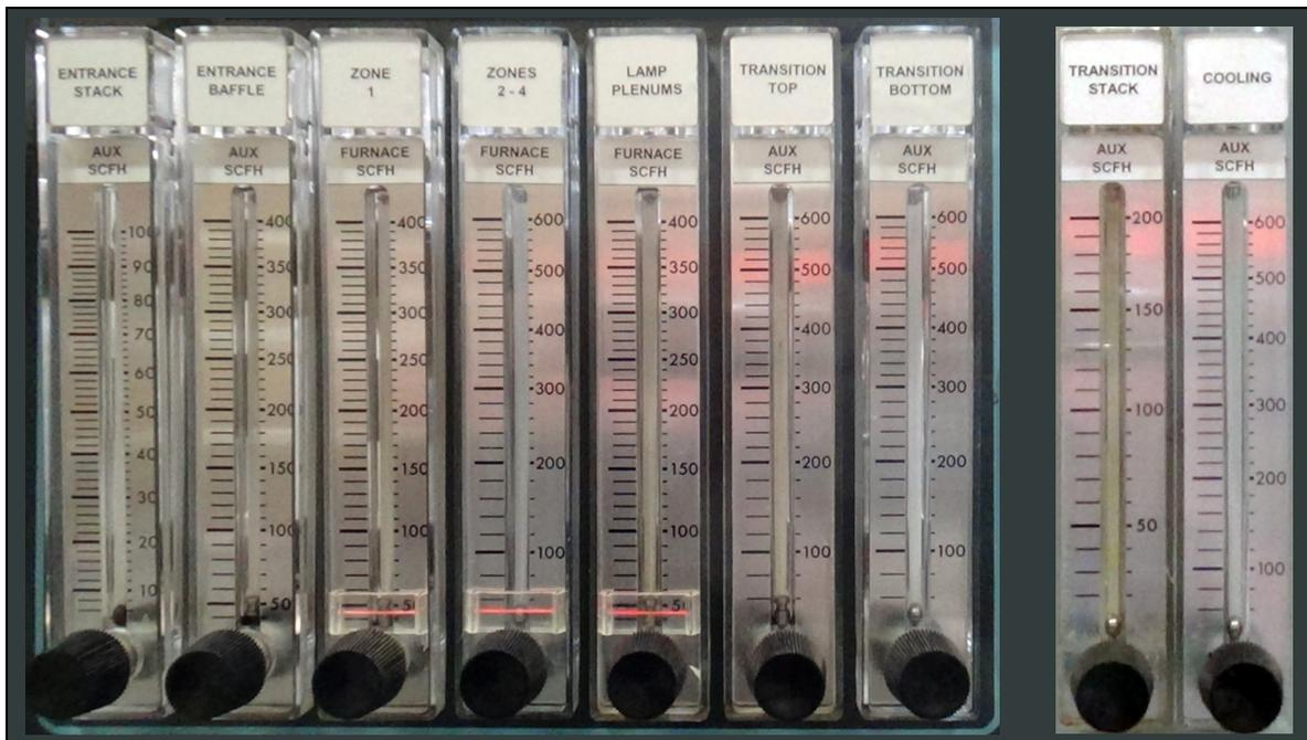
Figure 1-11 Gas Flowmeters - Dual Mode
