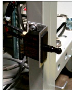
Panel Switch Installed - Bypass Mode Position
