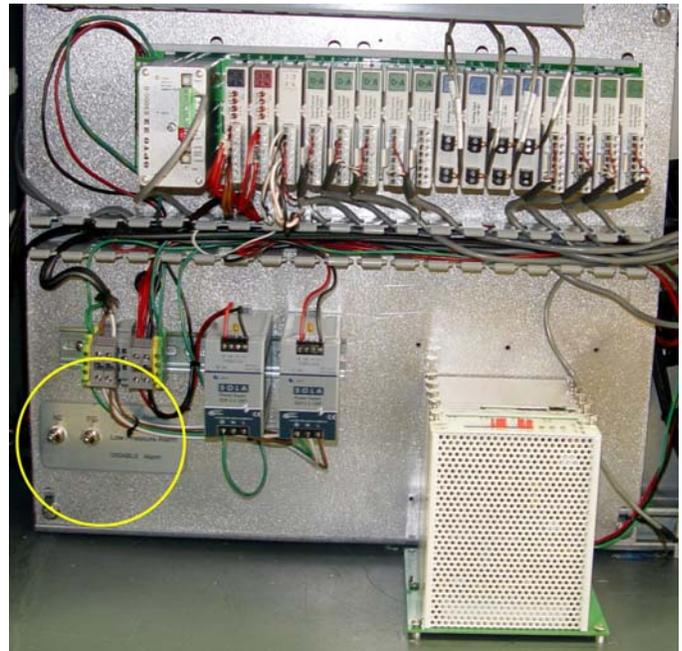
Figure 3.14.1 IPS Inlet Pressure Switch
