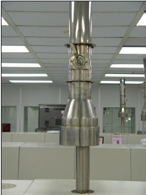
Figure 1.2.11 Exhaust Connection
