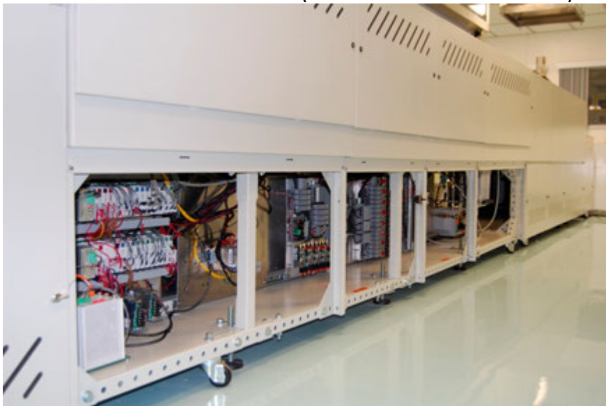
S-1209XH Furnace on Site with Lower Panels removed (3250 mm L x 960 mm W x 1700 mm H, (240 mm belt)
