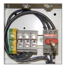
Figure 1-18 Disconnect Switch and Power Connection Terminal Blocks
