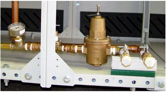
Figure 1-30 CAWC Water Supply & Drain Connections
