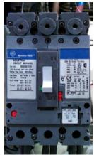
Figure 1-15 Circuit Breaker detail
