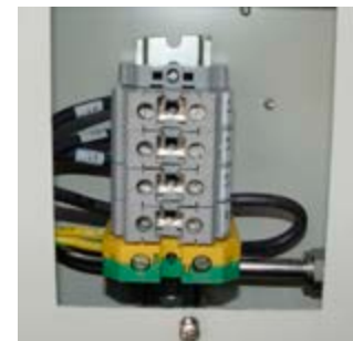
Figure 2-16 380-415Vac, 3PH 4-wire
