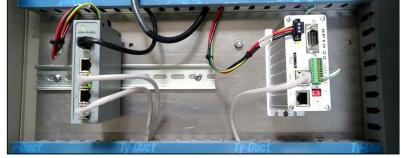
Figure 1-17 Ethernet Switch (L) & Controller (R)
