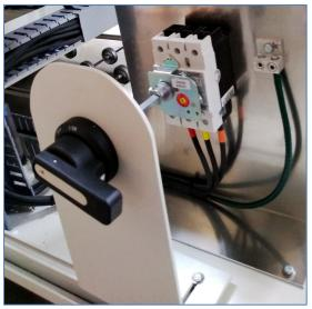
Figure1-25 3-Ph Circuit Breaker-Panel OFF
