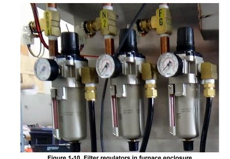
Figure 1-10 Filter regulators in furnace enclosure
