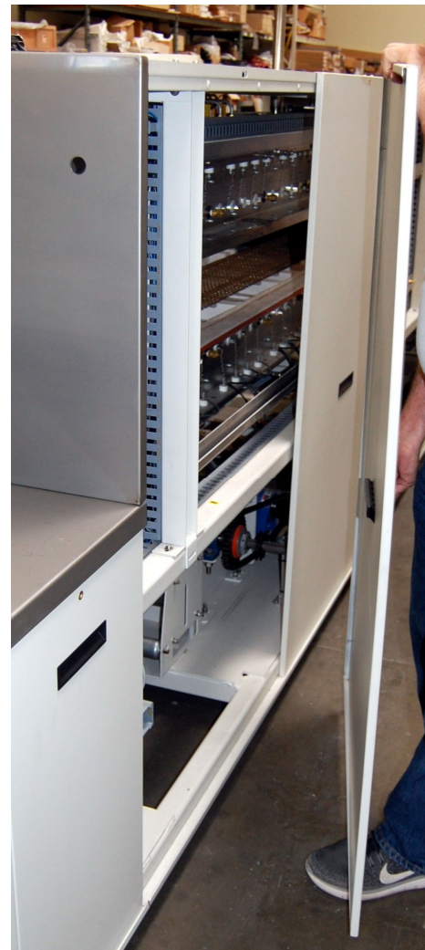
Figure 4-10 Remove panel and place in safe location
