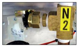
Figure 3-56 IPS Inlet Pressure Switch
