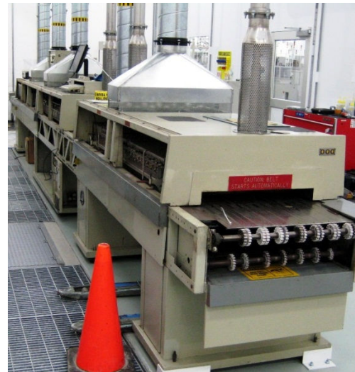
Figure 2-28 Cabinet Exhaust Examples
