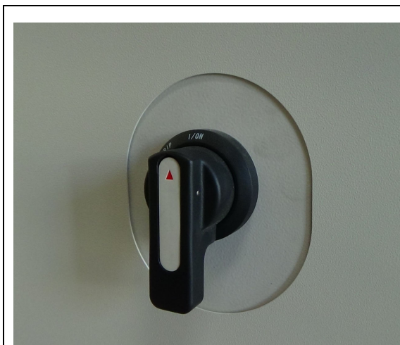
Figure 1-23 3-Phase Circuit Breaker
