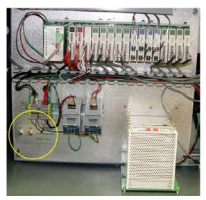
Figure 3-7 IPS Inlet Pressure Switch Location
