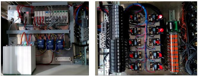
Figure 3-2 Power Distribution and Safety panels
