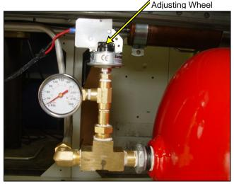
Figure 3-35 Air Pressure sensor
