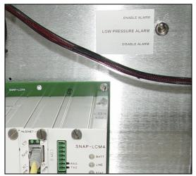
Figure 3-34 Enable Low Pressure Alarm switch
