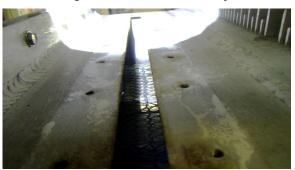
Figure 4-47 Transition Tunnel Stack Orifice Plate
