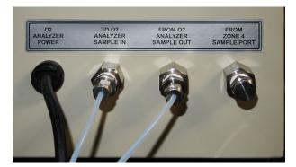
Figure 2-41 OA furnace control enclosure connections
