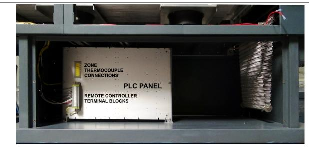
Figure 2-43 PLC Panel and Remote Connections
