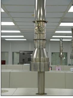
Figure 2-31 Exhaust Connection
