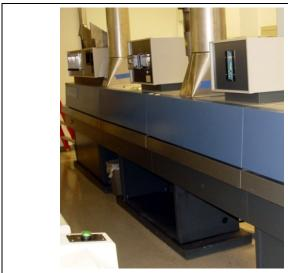
Figure 2-35 Cabinet Exhaust Example
