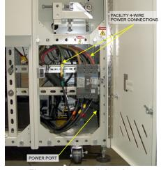
Figure 2-25 Circuit Breaker panel
