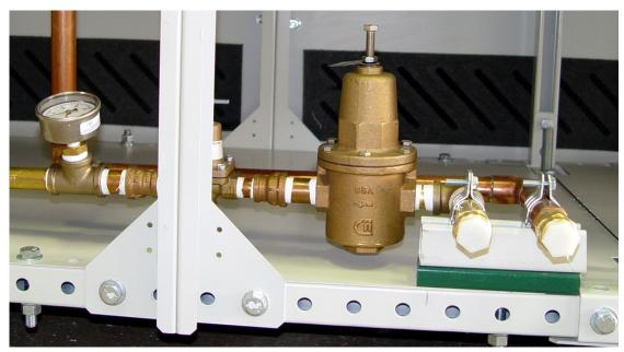
Figure 2-45 CAWC Water Supply & Drain Connections
