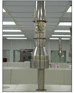
Figure 2-25 Exhaust Connection
