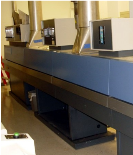
Figure 1-33 Cabinet Exhaust Example
