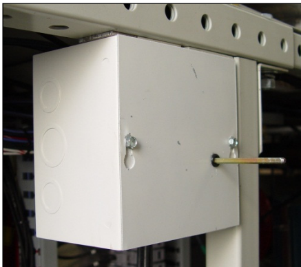
Figure 1-22 Interlock disconnect switch enclosure
