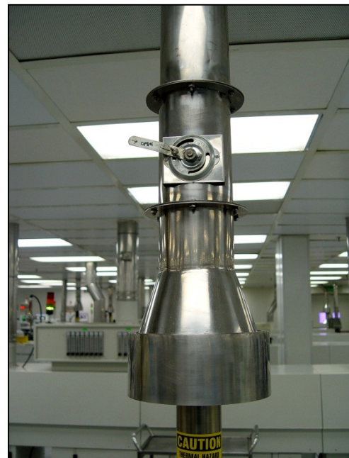
Figure 1-32 Exhaust Connection Detail
