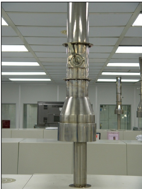
Figure 1-31 Exhaust Connection
