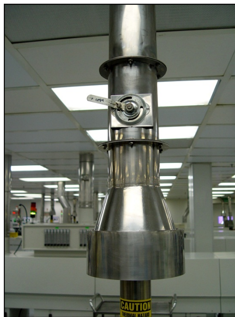
Figure 1-32 Exhaust Connection Detail
