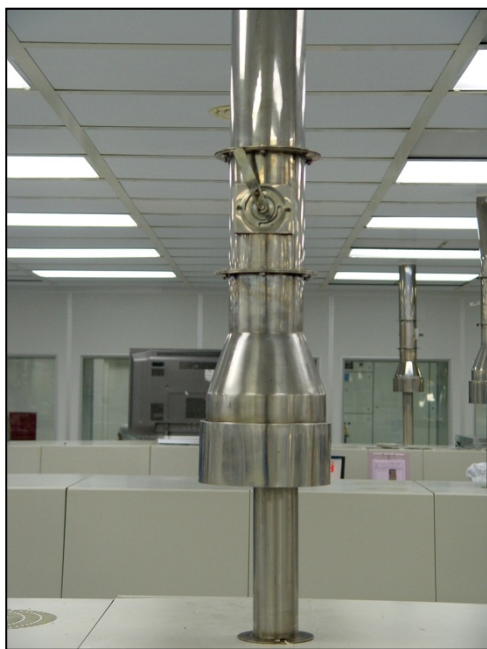
Figure 1-31 Exhaust Connection
