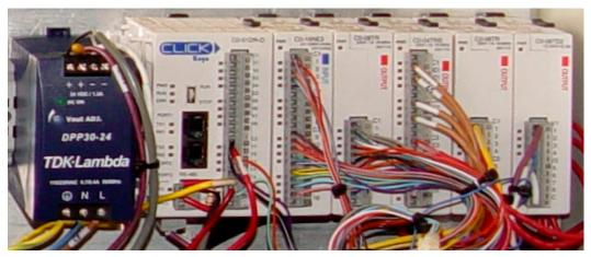
Figure 1-22 PLC and Power Supply
